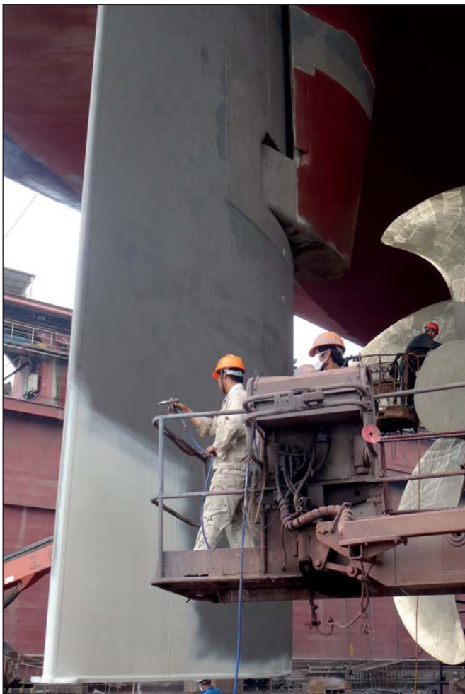
Only minor touch-ups will be needed during future drydockings.
