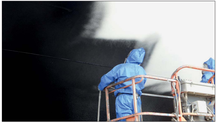
Application of second layer on ferry in Canada.
