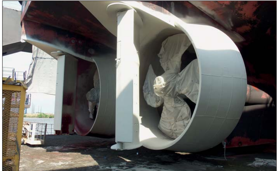
Rudders and propeller nozzles of tug after application of first layer.
