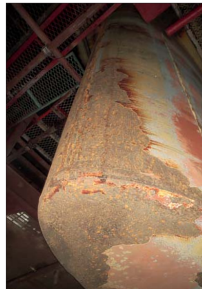
Rudders can suffer from corrosion damage much worse than this if not protected properly.
