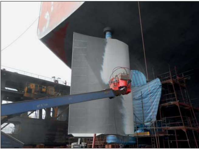
Application of first layer of Ecoshield.
