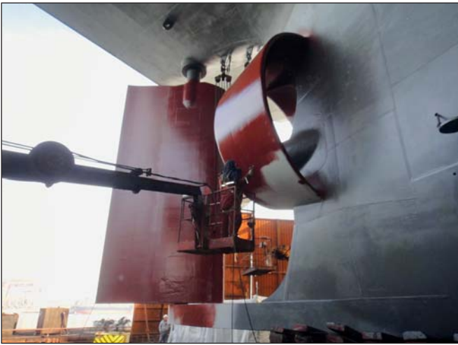
Application of second layer of Ecoshield on nozzle.
