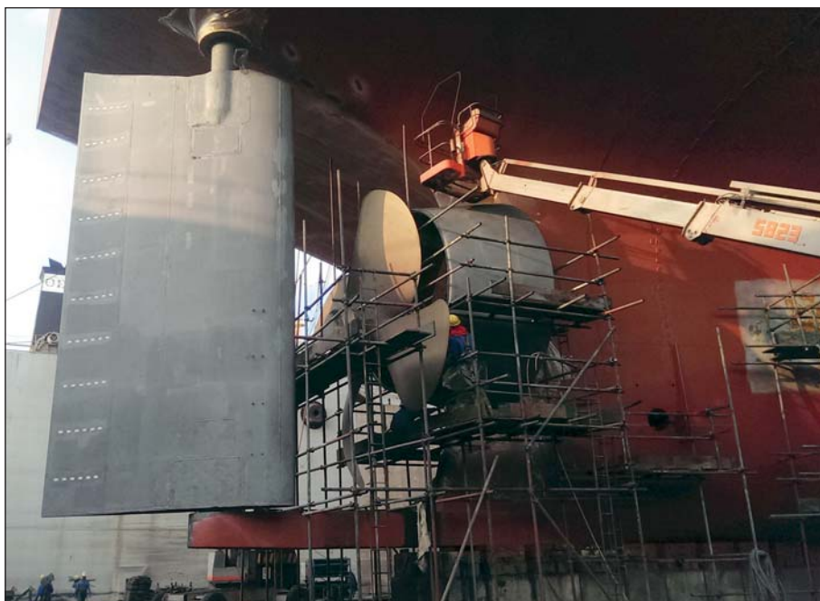
Rudder after surface preparation.
