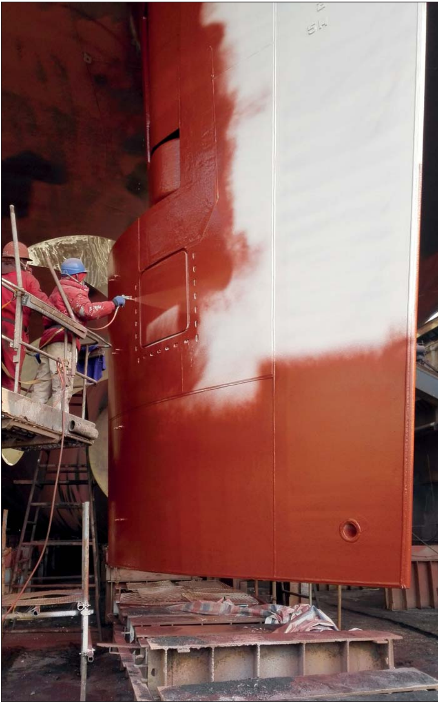
Ecoshield is applied in only two layers.
