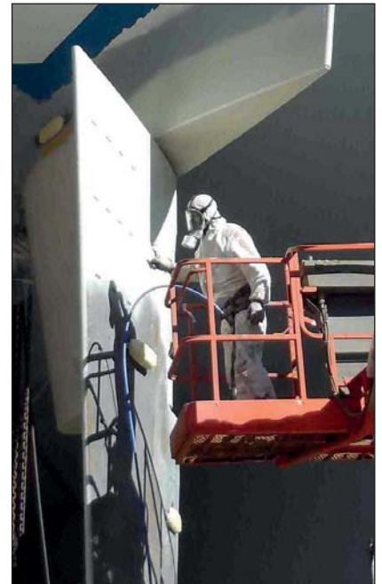
Ecoshield is applied in two identical layers.
