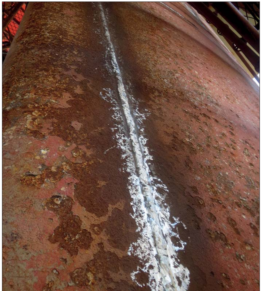
The effect of cavitation damage can be devastating if a rudder is not protected properly.
