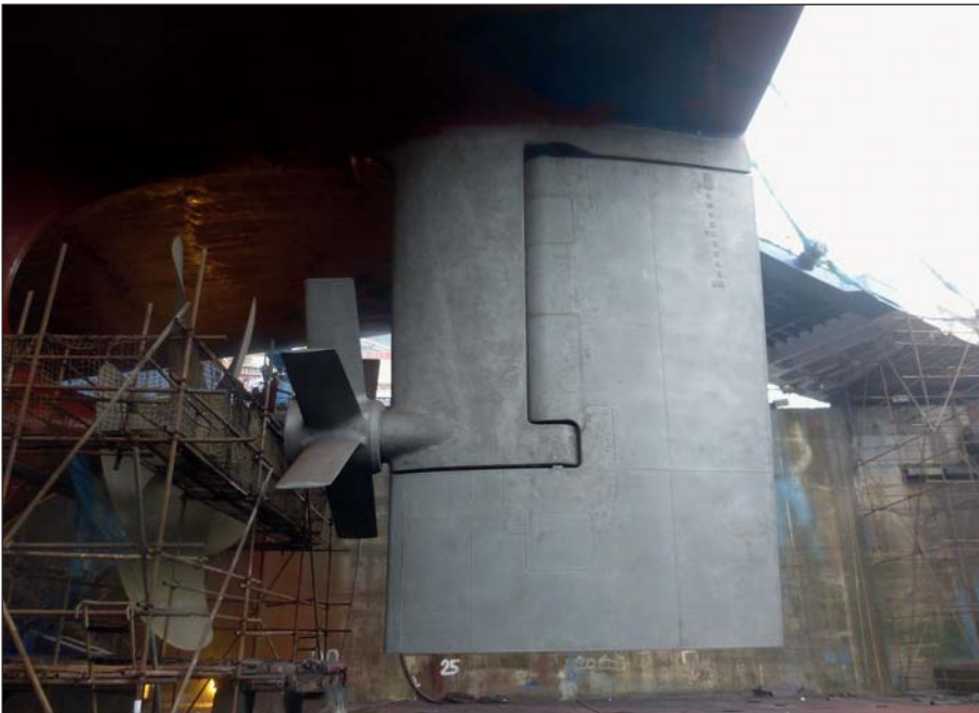
Surface preparation prior to Ecoshield application.
