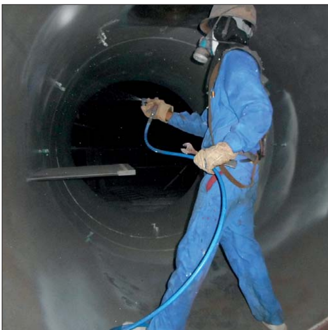
Thruster tunnels and other running gear can also be protected with Ecoshield.
