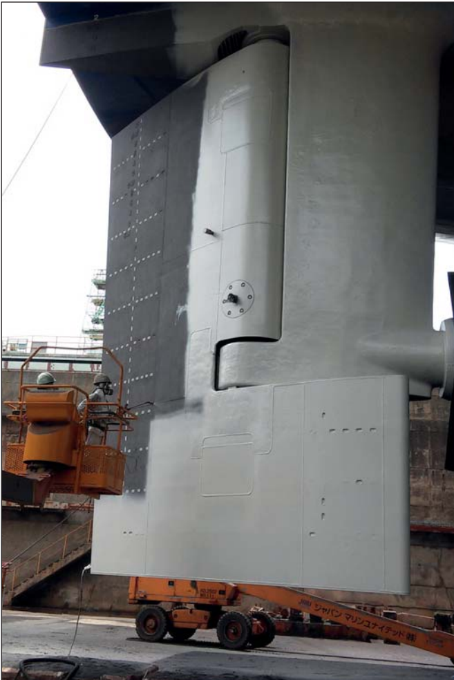
Application of first of two identical Ecoshield layers.
