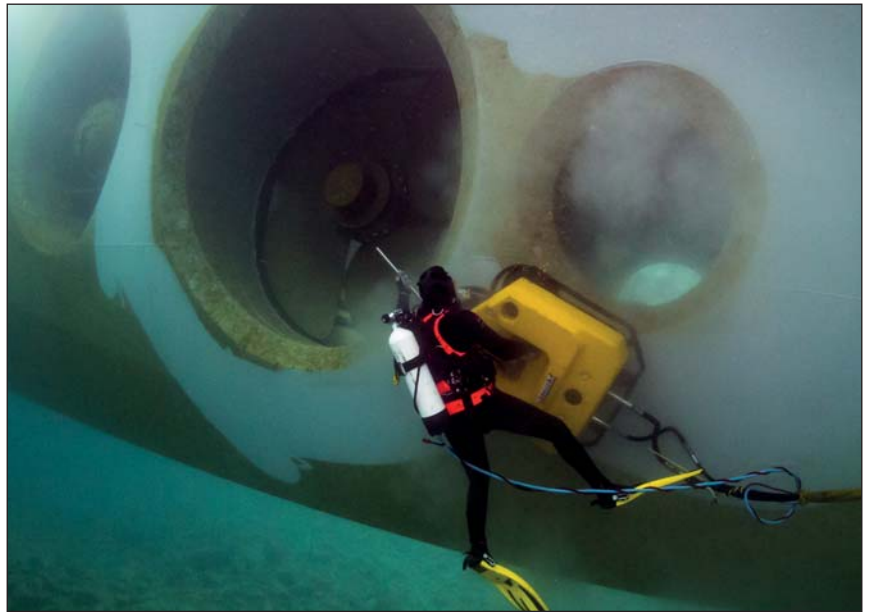
Routine in-water cleaning keeps this cruise ship's Ecospeed coated hull clean. In fact Ecospeed gets a little smoother with each cleaning.
