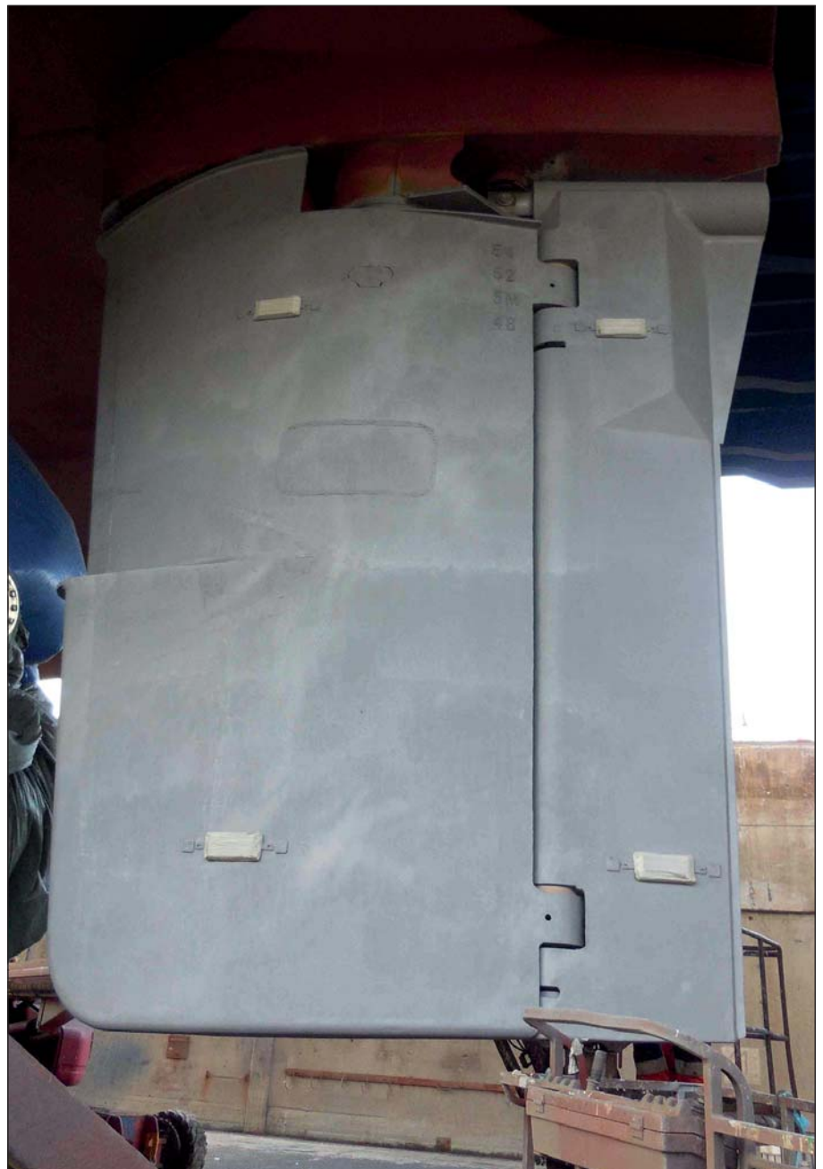
Surface preparation prior to Ecoshield application.
