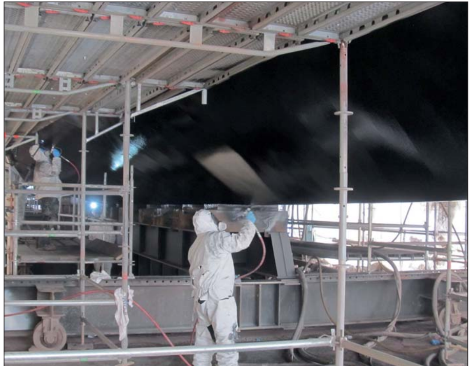
Application of smaller vessels can be done in a single day.
