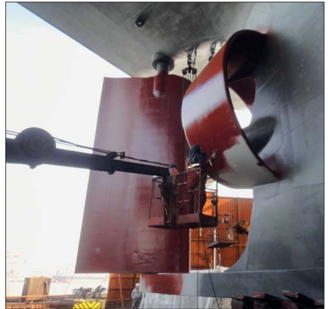
Application of the second layer of Ecoshield on nozzle.
