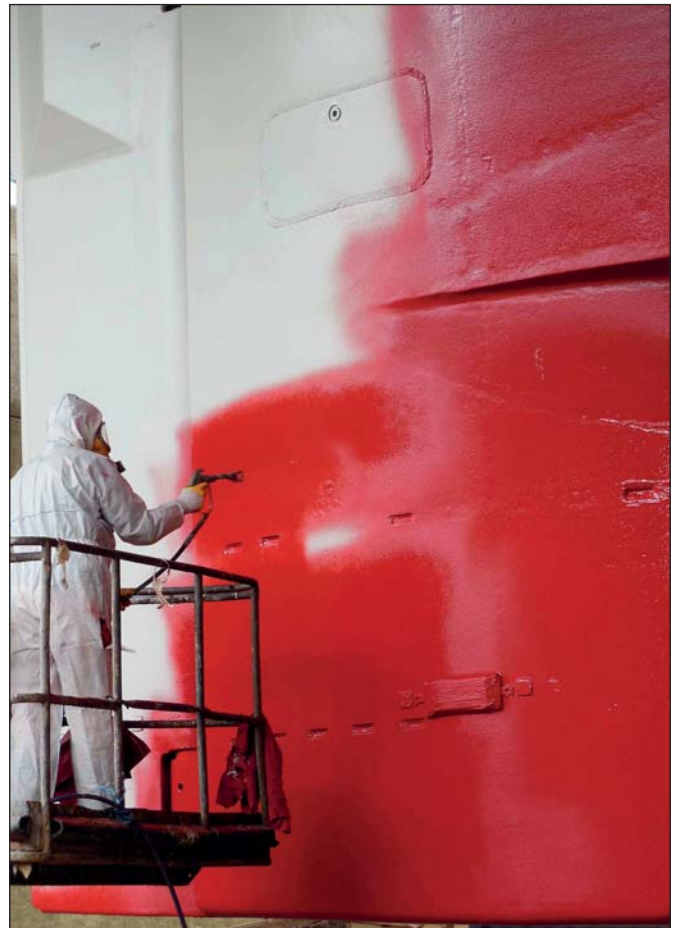
Overcoating time in between layers can be as short as three hours.
