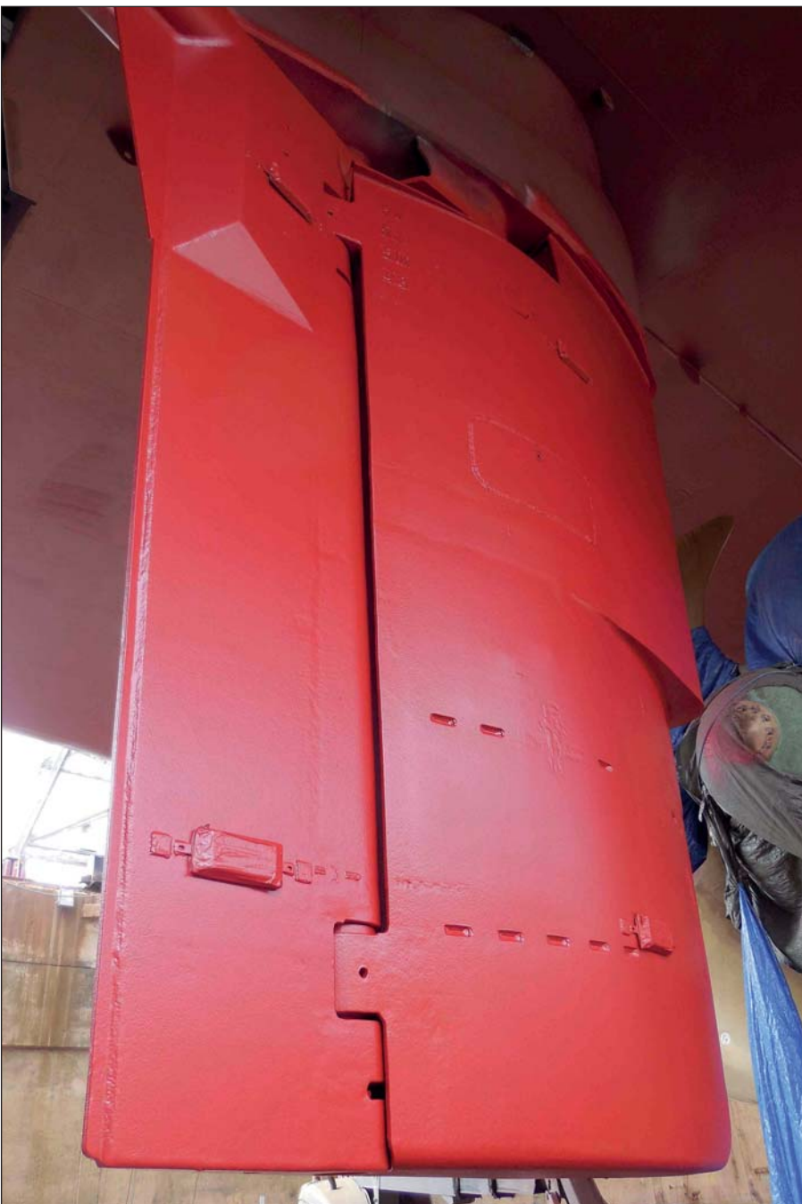
No further corrosion or pitting damage will appear on these rudders.
