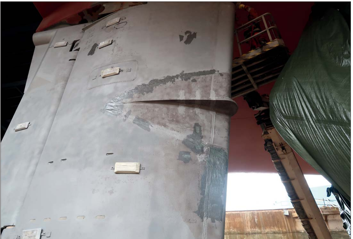
The rudder is now ready for Ecoshield application.
