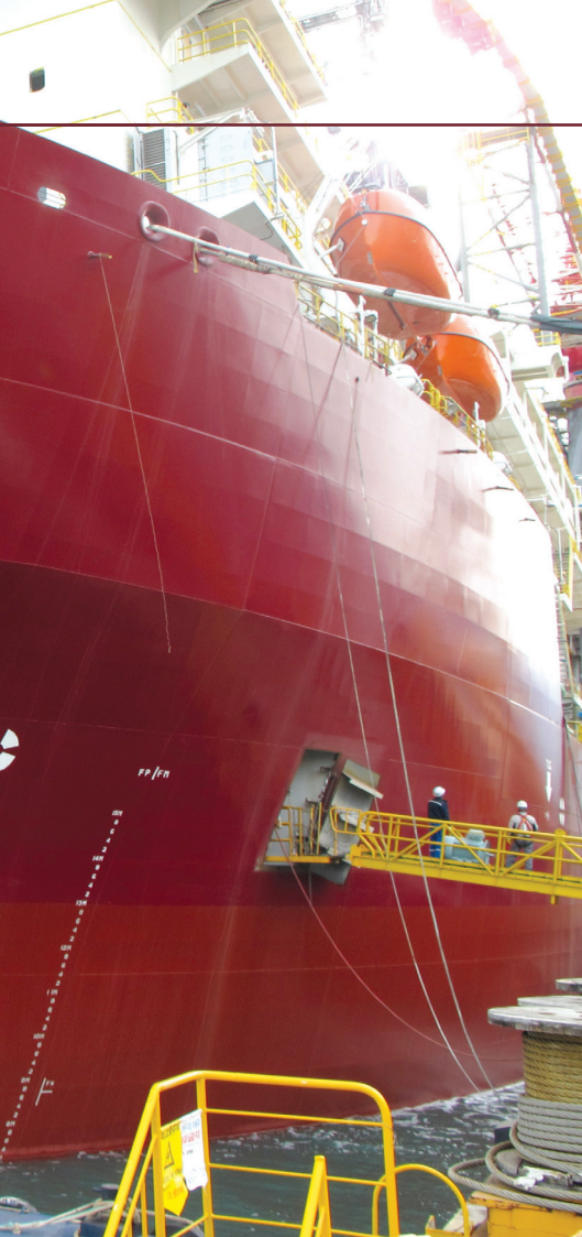
Sigma Nexeon 750 antifouling on one of Odebrecht Oil and Gas' newbuild drillships after a long outfitting period
