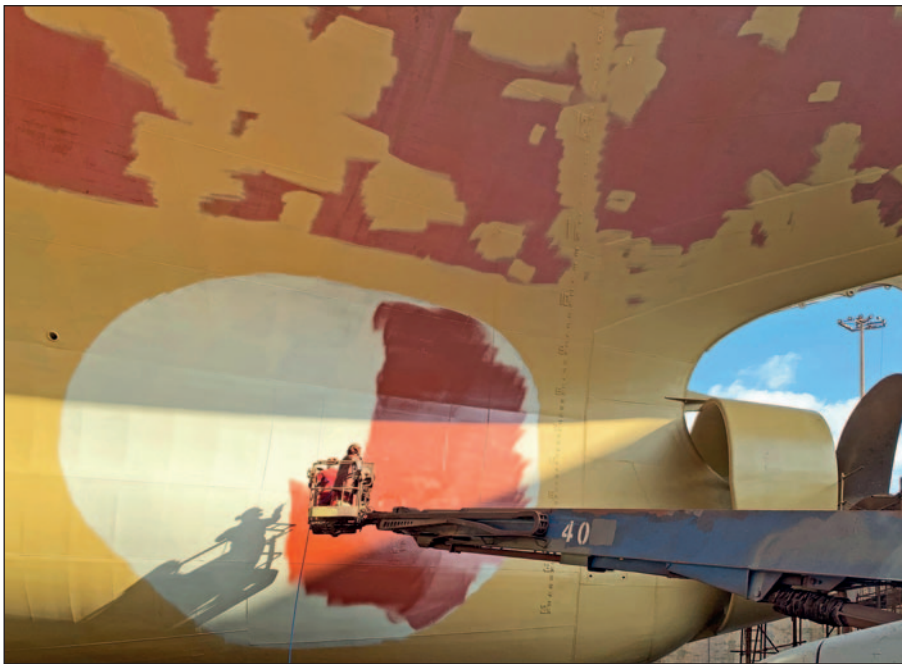
Ecospeed will protect the area around the scrubber outlets for the ship's entire lifetime.
