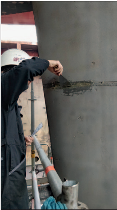
Applying Ecofix on the pitted areas of a rudder.
