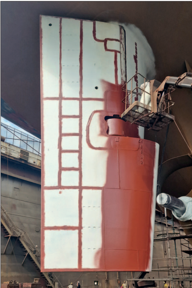
The second layer can be applied as soon as three hours after the first.
