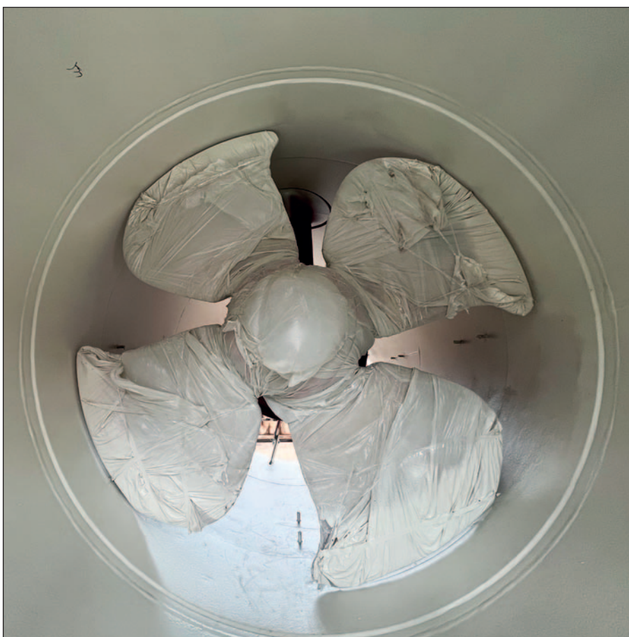
Thruster tunnel after the first Ecoshield layer was applied.
