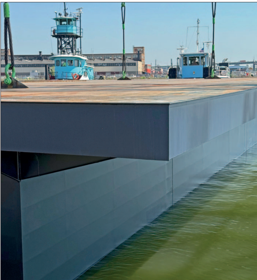
Detail: shell of pilot + POOL with Ecolock coating, Just lifted into water at Port Newark, 30 July 2025. (Image from Friends of + Pool)
