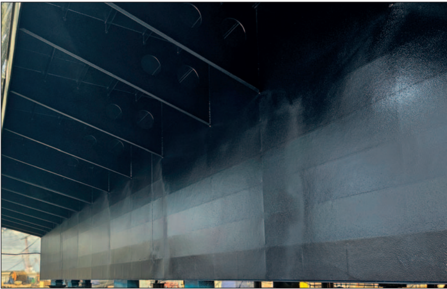
The first and second coat combined create a dry film thickness (DFT) of at least 1000 microns (40 mil).
