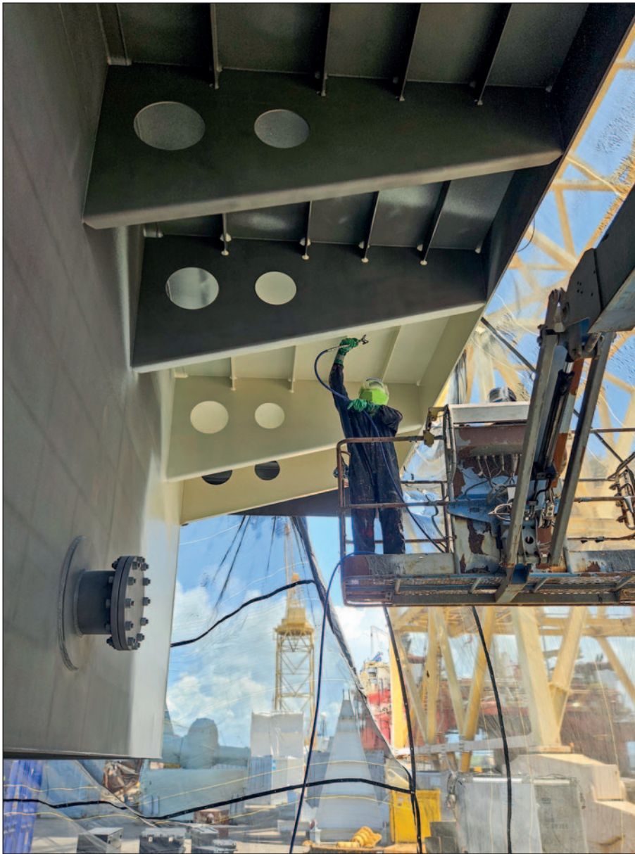
Application of first coat of Ecolock directly to the grit blasted steel by USA DeBusk at Bollinger Shipyards.
