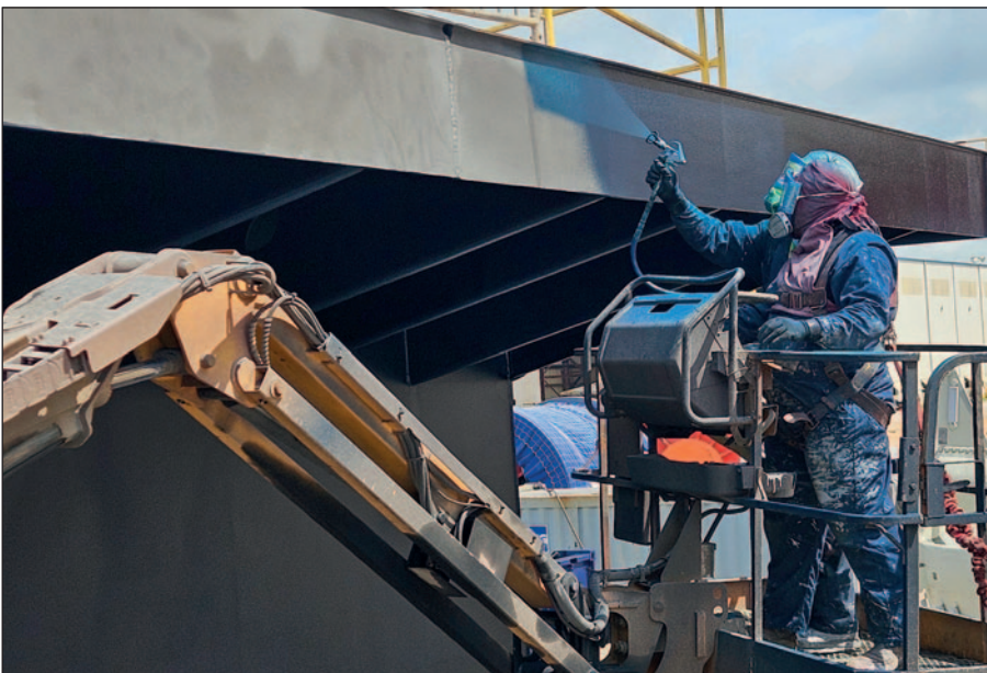
Finishing application of the second coat of Ecolock.
