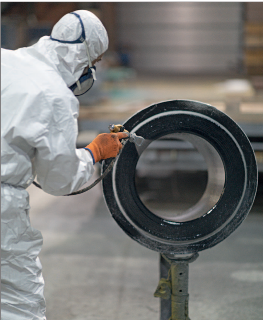
Ecospeed application on scrubber pipe.
