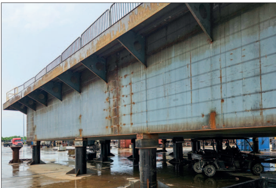
The first test pool shell after construction at Bollinger Shipyards, prior to preparation for painting.
