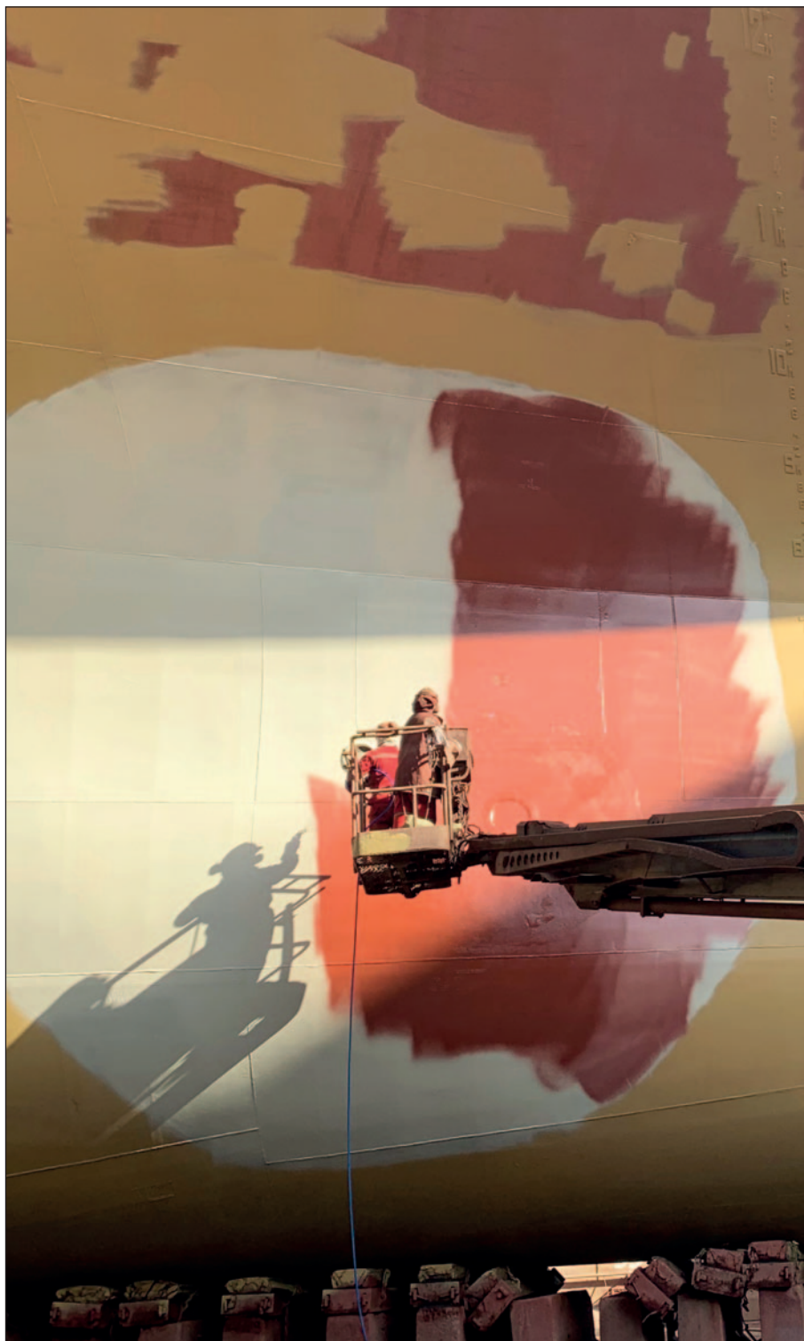
The second layer can be applied as soon as 3 hours after the first.
