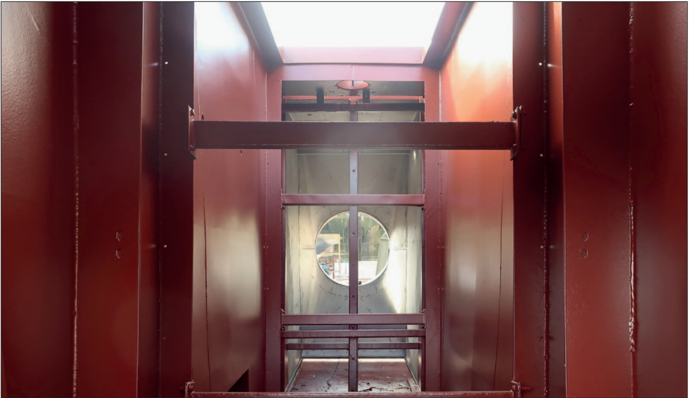
Inside of scrubber after application of second Ecospeed layer.
